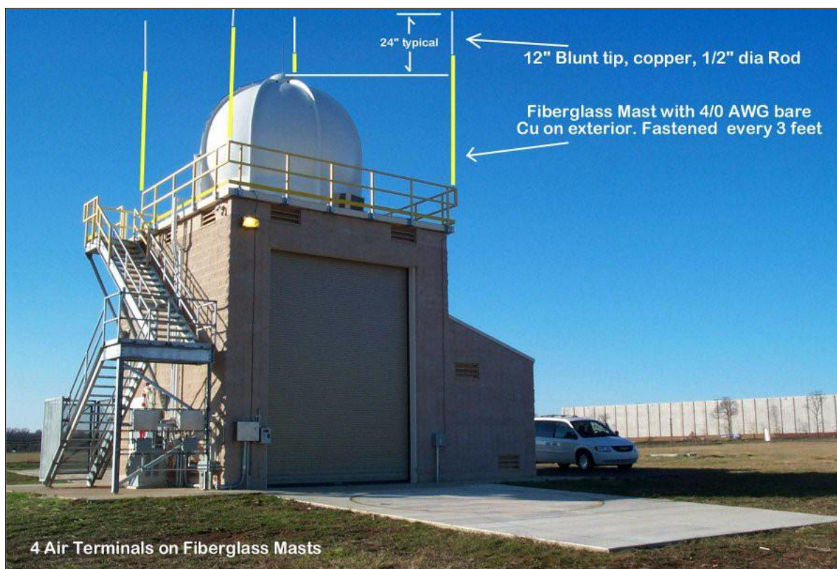
Figure 2-3. Lightning Protection for Upper Air Buildings (Franklin Rod Design)
